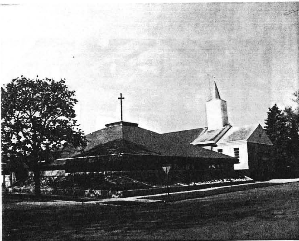
View from the corner of Church & Foote Streets
