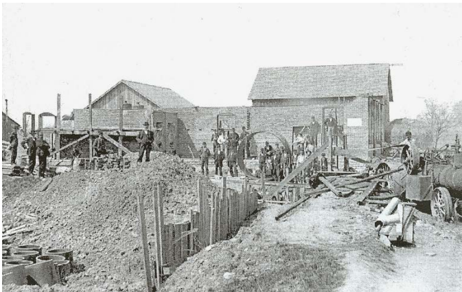
Construction of the City Water Works
